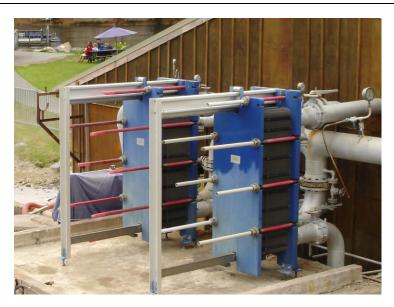
Figure 3.2. Plate heat exchanger at the Taupo Prawn farm (Thain et al 2006)
